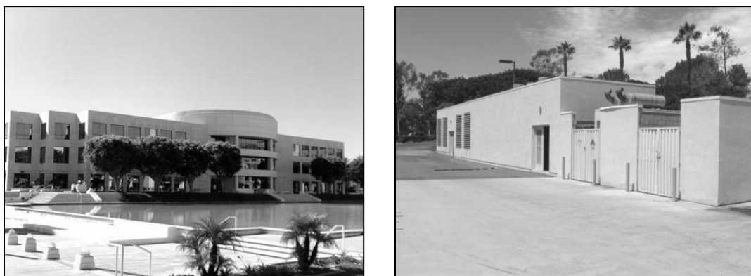
Figure 1: Photos of Amylin Building and Cooling Tower Mechanical Yard
