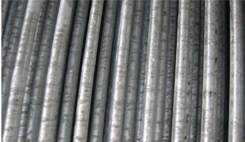
**Figure II – Counter Flow Tower Galvanized Tube Bundle**
